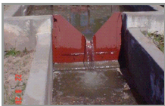
Figura II.20: Vertedero triangular
